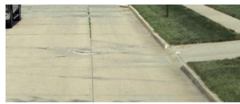
Figure 19: Example of "Poor" Condition (PCC) – North 17<sup>th</sup> Street
