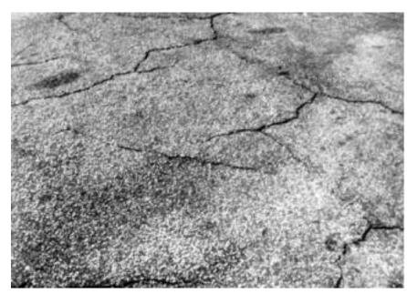
Figure 6: Example of Block Cracking (ASTM)
