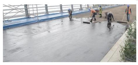
Figure 30: Slurry Seal Being Placed by Hand (Miraflores)
