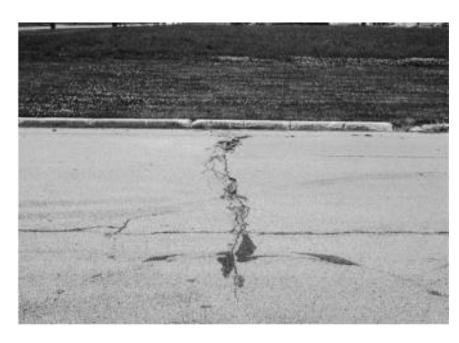
Figure 8: Example of Transverse Crack (ASTM)
