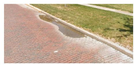
Figure 40: Area Distortion of Rapids Street Holding Water
