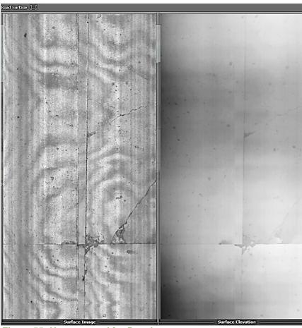
Figure 55: Unaccounted for Punchout
