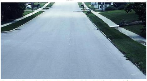
**Figure 12: Example of "Very Good" Condition (HMA) – South 14<sup>th</sup> Street**This picture was taken from the 2021 data collection records. South 14<sup>th</sup> St near Greene has a very high PCI of 92 /100 because it demonstrates no visible pavement distresses. Likely because it was overlayed recently.
