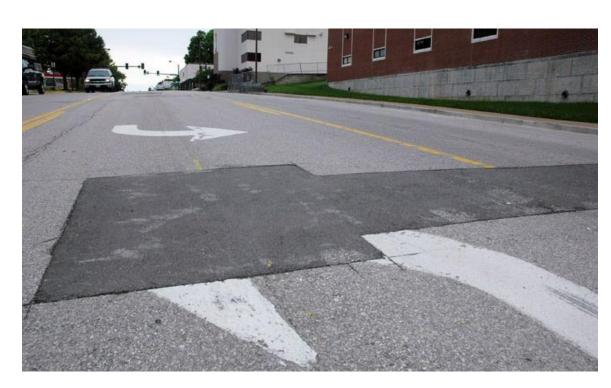
Figure 37: HMA Patching with Localized Pavement Removal (KOMU)
