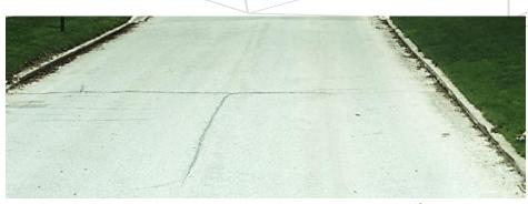
Figure 14: Example of "Good" Condition (HMA) – North 15<sup>th</sup> Street
