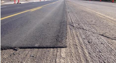
Figure 28: HMA Overlay Placed On Milled Pavement (Famartin)
