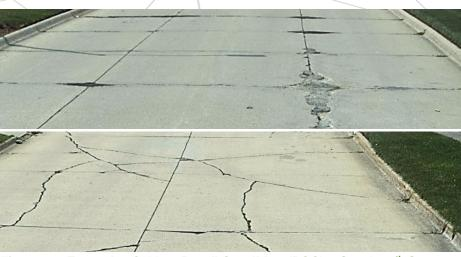
Figure 22: Example of "Very Poor" Condition (PCC) – South 16<sup>th</sup> Street
