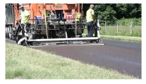
Figure 31: Microsurfacing Crew at Work. (Eric Pulley).
