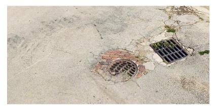
Figure 41: Evidence of Brick Street Under a 30-year old Overlay
