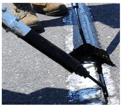
Figure 36: Crack Sealing Performed W/ Routing (USAF/Kenna Jackson)
