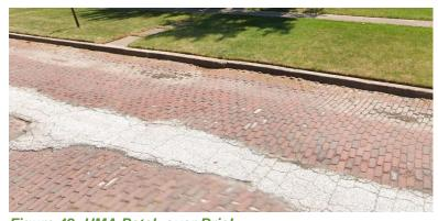
Figure 42: HMA Patch over Brick
