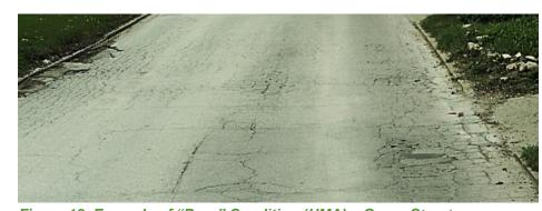
Figure 18: Example of "Poor" Condition (HMA) – Grove Street
