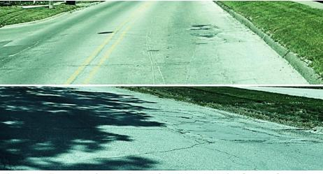
Figure 20: Example of "Very Poor" Condition (HMA) – Greene Street
