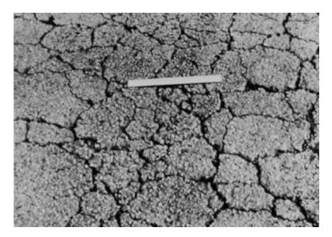
Figure 5: Example of Alligator Cracking (ASTM)
