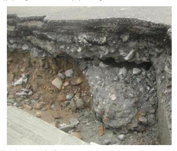
Figure 61: Under Pavement Voiding (Chen)
