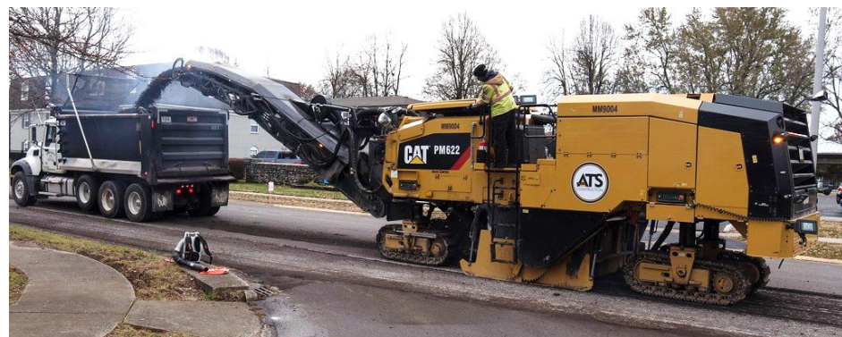
Figure 29: Cold Milling Machine (Anthony Neff) Cold Milling Machines like the Caterpillar PM 622 above are used to strip off the top layer of pavement. Those millings could then be used for in-place recycling, or the pavement could receive a new 3” overlay.
