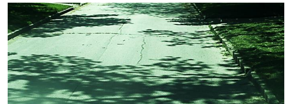
Figure 16: Example of “Fair” Condition (HMA) – Chance Court This image of Chance Ct is an example of HMA pavement in “Fair” condition, with a PCI of 50/100. There are very noticeable distresses but they only impact drivers slightly.
