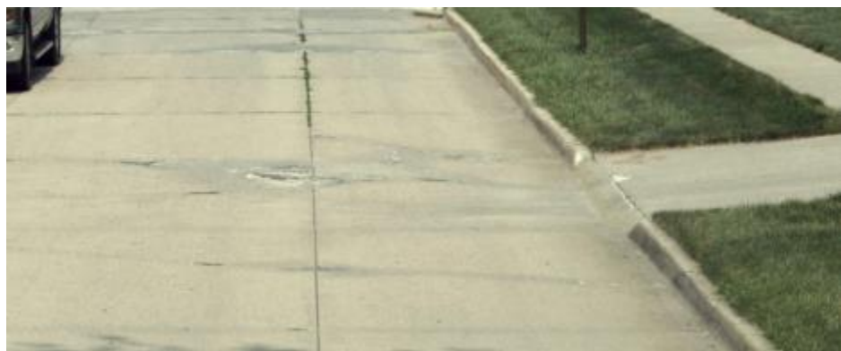
Figure 19: Example of "Poor" Condition (PCC) – North 17 th Street This image is an example of a PCC pavement in "Poor" condition. In 2021, the section of N 17 th St shown had a PCI of 26/100 due to joint failures.
