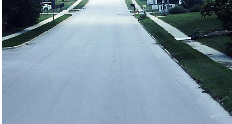
Figure 12: Example of “Very Good” Condition (HMA) – South 14 th Street This picture was taken from the 2021 data collection records. South 14 th St near Greene has a very high PCI of 92 /100 because it demonstrates no visible pavement distresses. Likely because it was overlaid recently.
