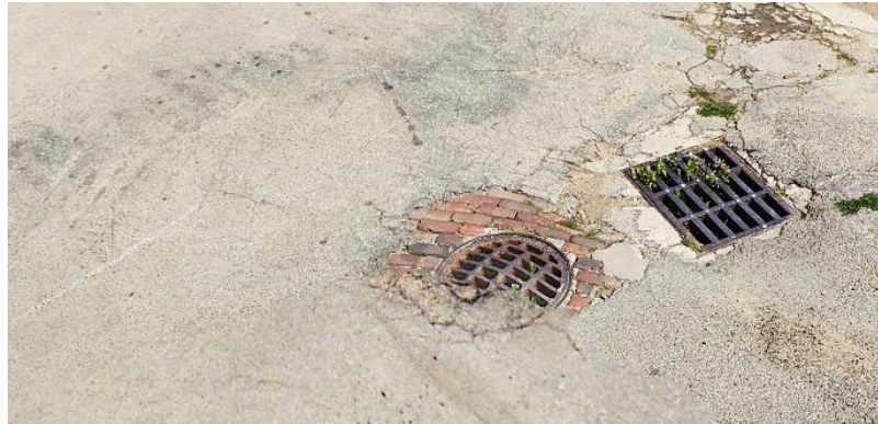
Figure 41: Evidence of Brick Street Under a 30-year old Overlay This photo from Anamosa shows an older brick street underneath an asphalt overlay.
