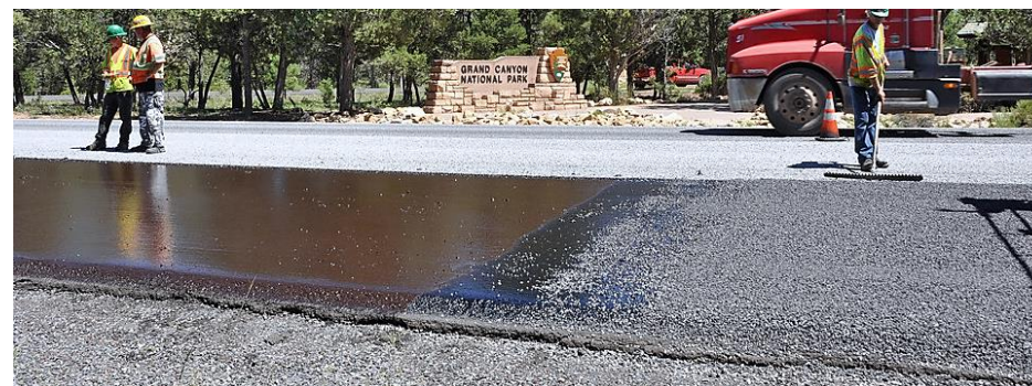
Figure 35: Cape Seal (Michael Quinn-NPS) This picture taken by the National Parks Service near the entrance to Grand Canyon National Park shows a loose chip seal (right) that is having a slurry seal applied (left) to effectively turn it into a cape seal.
